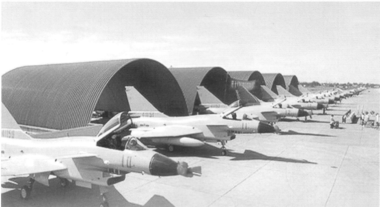
Fig.1 Roofing structures K-span arch
